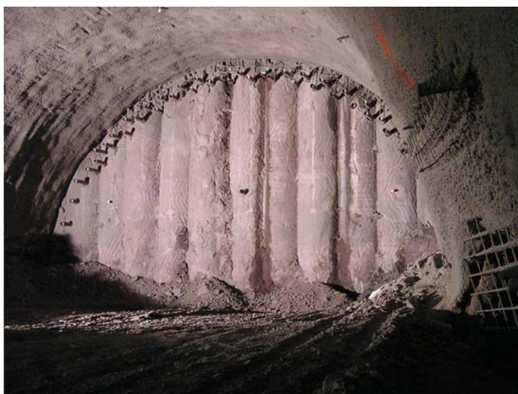
Figure 8: Umbrella from micropiles embedded into pile wall
